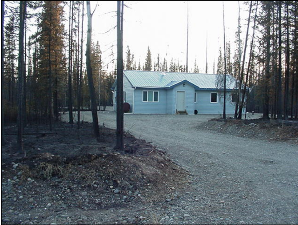
This structure had a 30' clearing down to mineral soil/gravel and metal siding.
