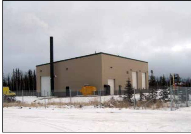
Left: The building that houses the woodchip-fired boiler and its equipment-under construction. Right: The completed facility. Photos: DOF
