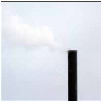
Steam released out of the boiler facility. Photo: DOF
