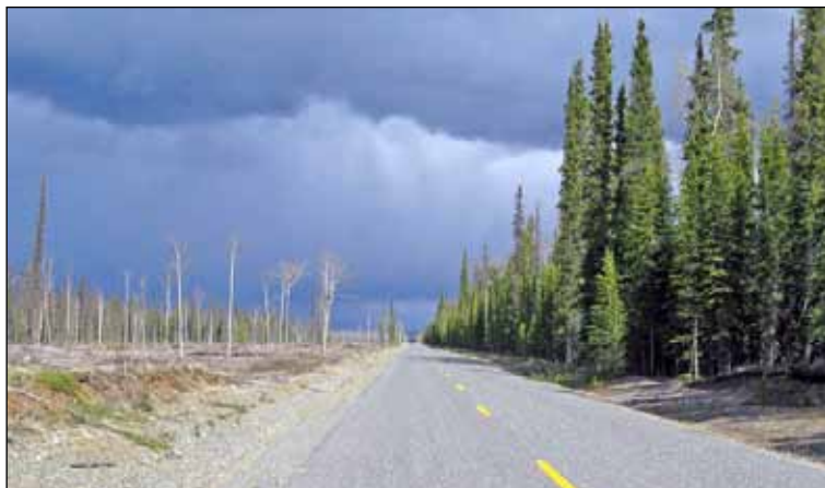
The road is a dividing line between a treated fuel reduction area on State land and the untreated forest on private land.
