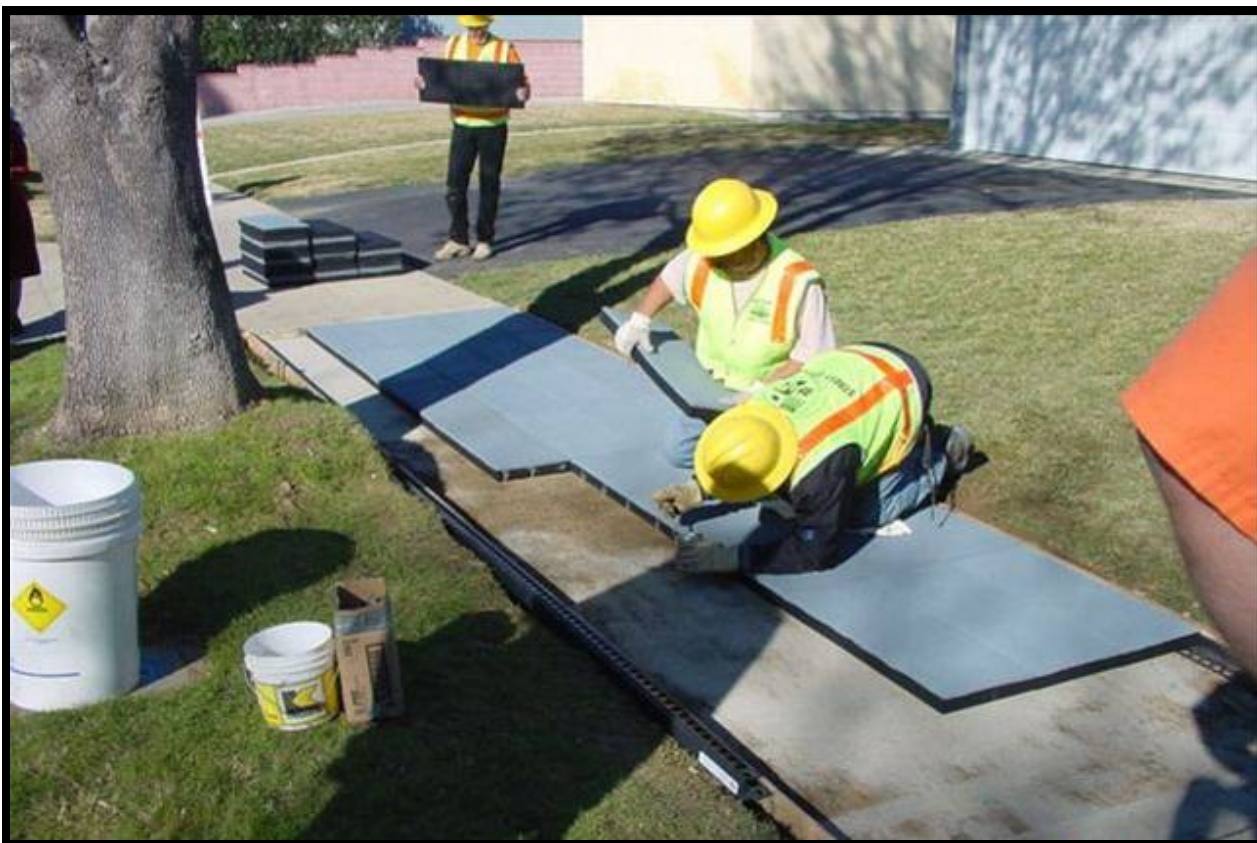
Figure 15 - Rubber sidewalk installation.
