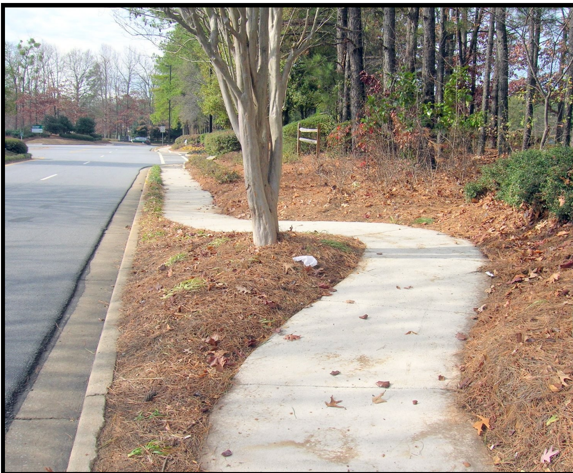
Figure 12 - Re-routing sidewalks around existing, large trees is a successful option.
