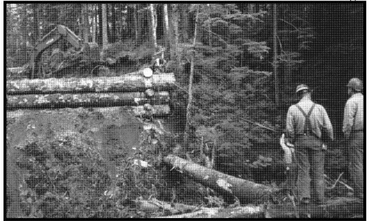
Log stringer bridge under construction in West Icy Bay. (Joel Nudelmann)
