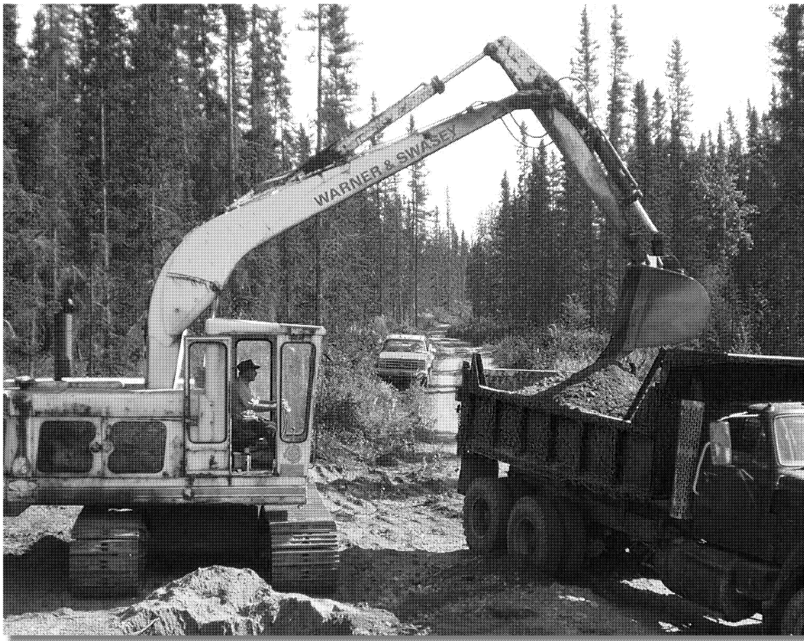
An excavator digs gravel to spread on a logging road for a Delta Area timber sale. The gravel was spread on road fabric covering the road bed. The 90-acre timber sale was purchased by Granite Mountain Alaska Lumber. (photo by Steve Joslin)
