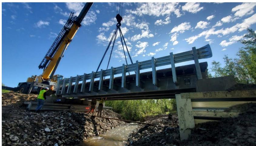
**Above:** Spring 2023, installation of the new Fortune Creek Bridge and abutments.
