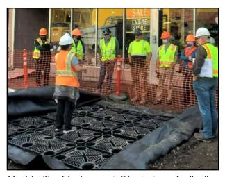
Municipality of Anchorage staff host a tour of soil cells being installed on 4<sup>th</sup> Avenue. The cells provide adequate soil for trees planted in sidewalk openings to reach mature sizes. (*Josh Hightower*)
