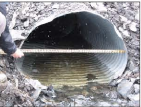
Stream culvert inspection
