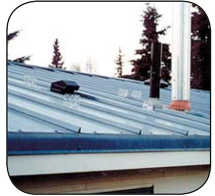
The most important step you can take to create a Firewise house is to build or reroof with a fire-resistant material such as a metal roof.
