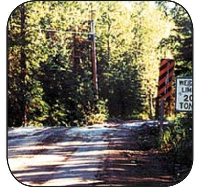
Roads, driveways, and bridges should be built to carry at least 40,000 pounds, which is the average weight of a fire engine.
