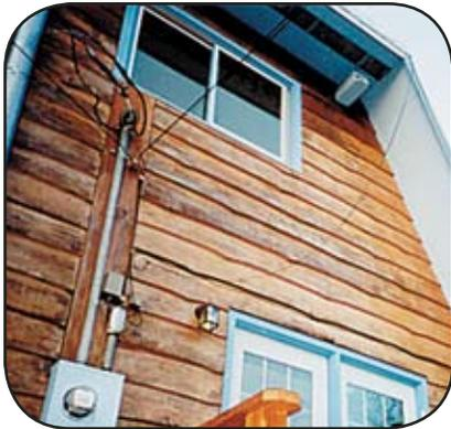
Roof eaves should be enclosed with fire-resistant materials and vents screened with  $\frac{1}{4}$ -inch nonflammable mesh screen.
