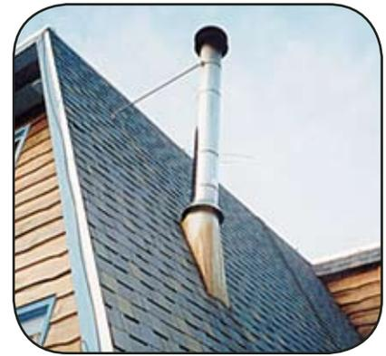
Every chimney and stovepipe must be covered with no larger than  $\frac{5}{8}$ -inch nonflammable screen.
