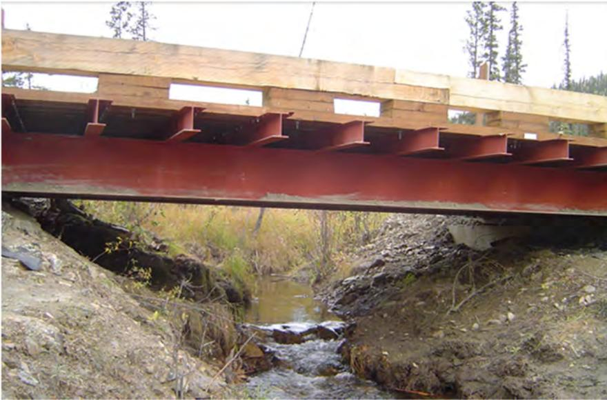
Figure 58. The Standard Creek bridge near the Tanana Valley State Forest is an example of installing a bridge instead of a culvert in a deep v-notch or drainage, in keeping with the Alaska Forest Resources and Practices Act. ©2020 ADOF
