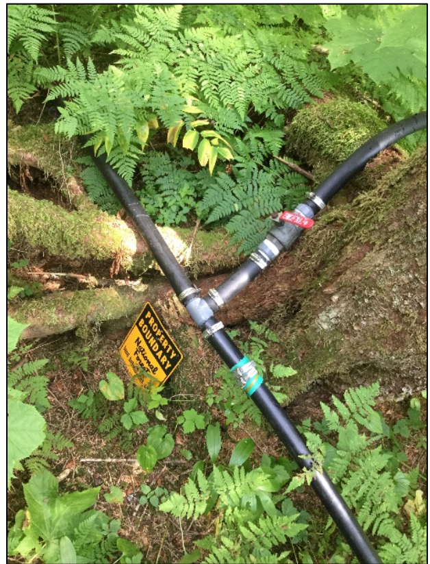
Photo 9. Maas waterline pipe junction.
