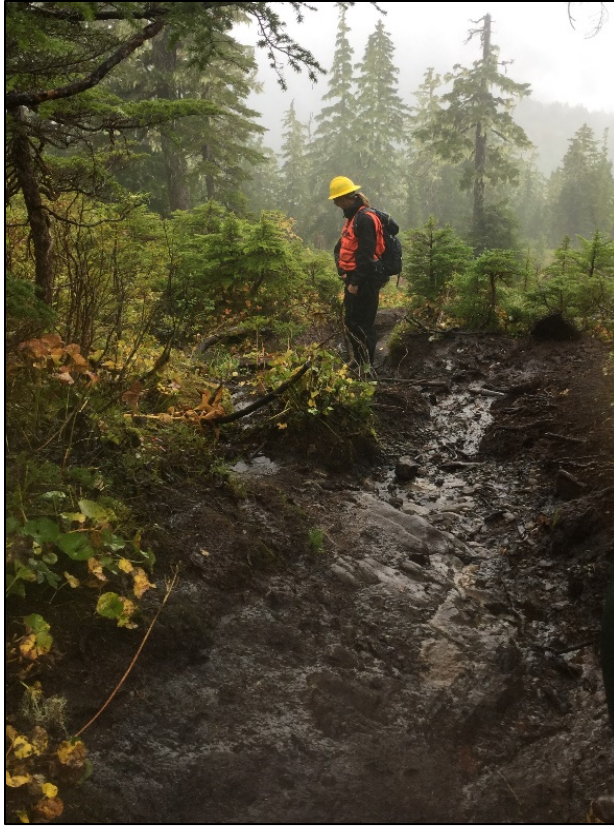
Photo 4. Rill-eroded section of evaluated trail segment.
